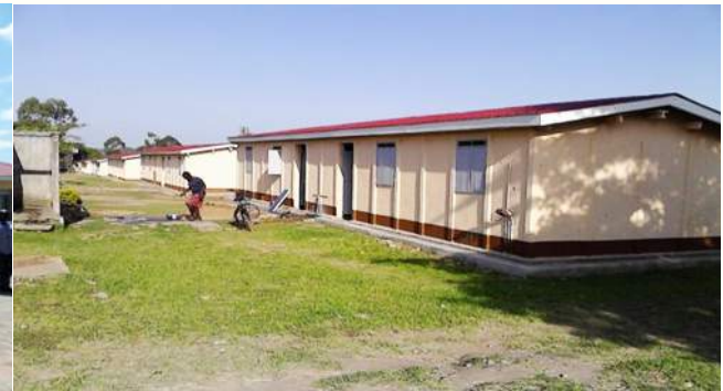
Renovated Barracks - Arua
