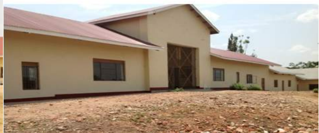
Renovation of Kitalya Administration block
