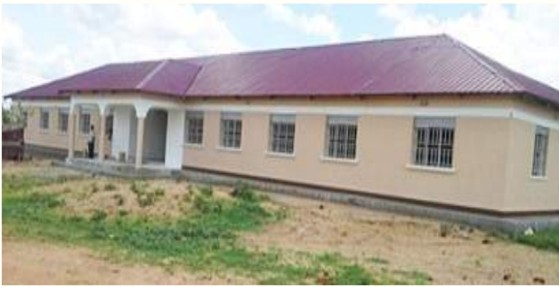
Kotido Police Station
