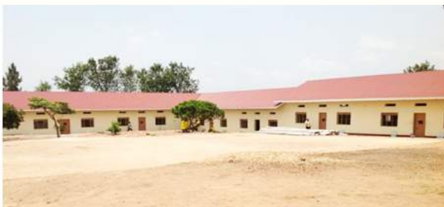
Kitalya Renovation of wards completed
